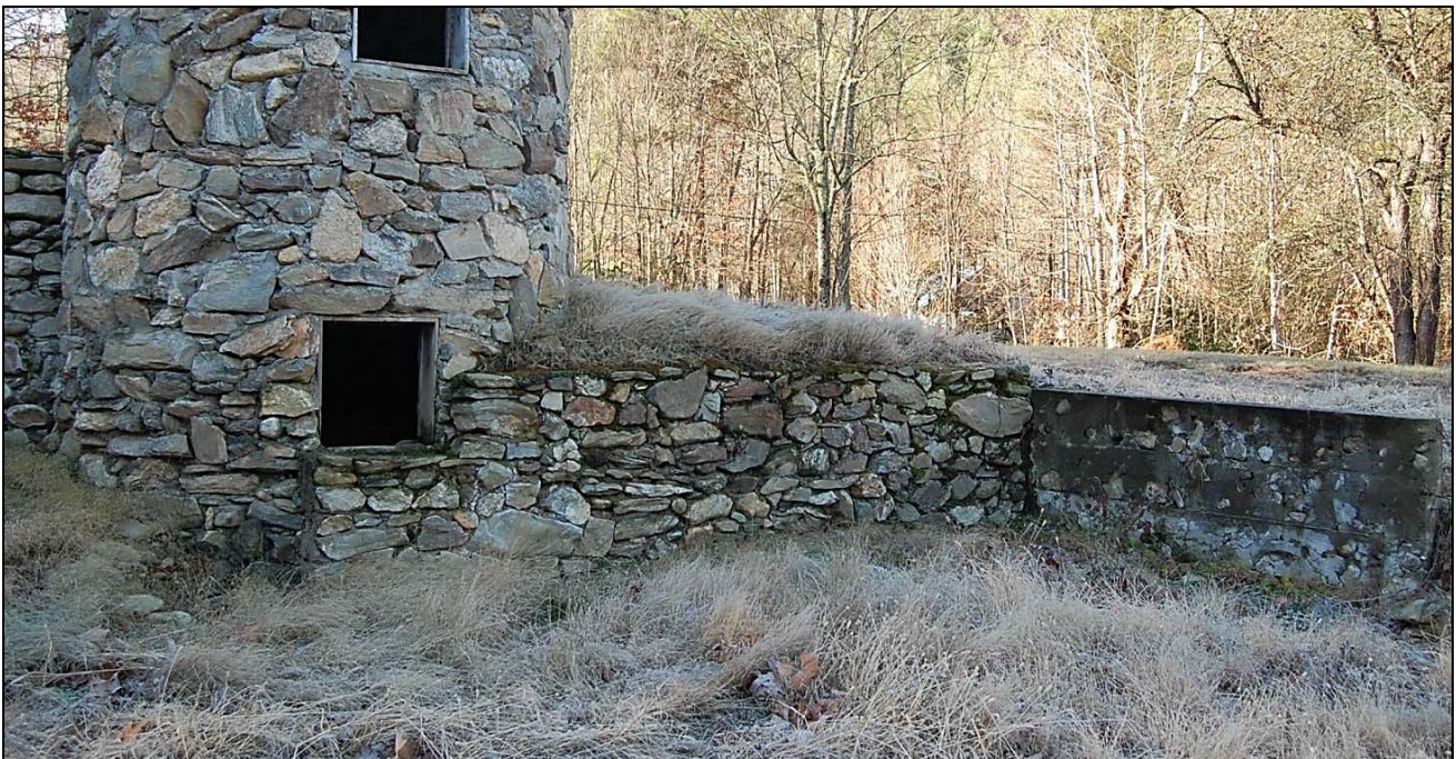
Figure 16. Looking southwest at three sections of foundation wall and west silo
