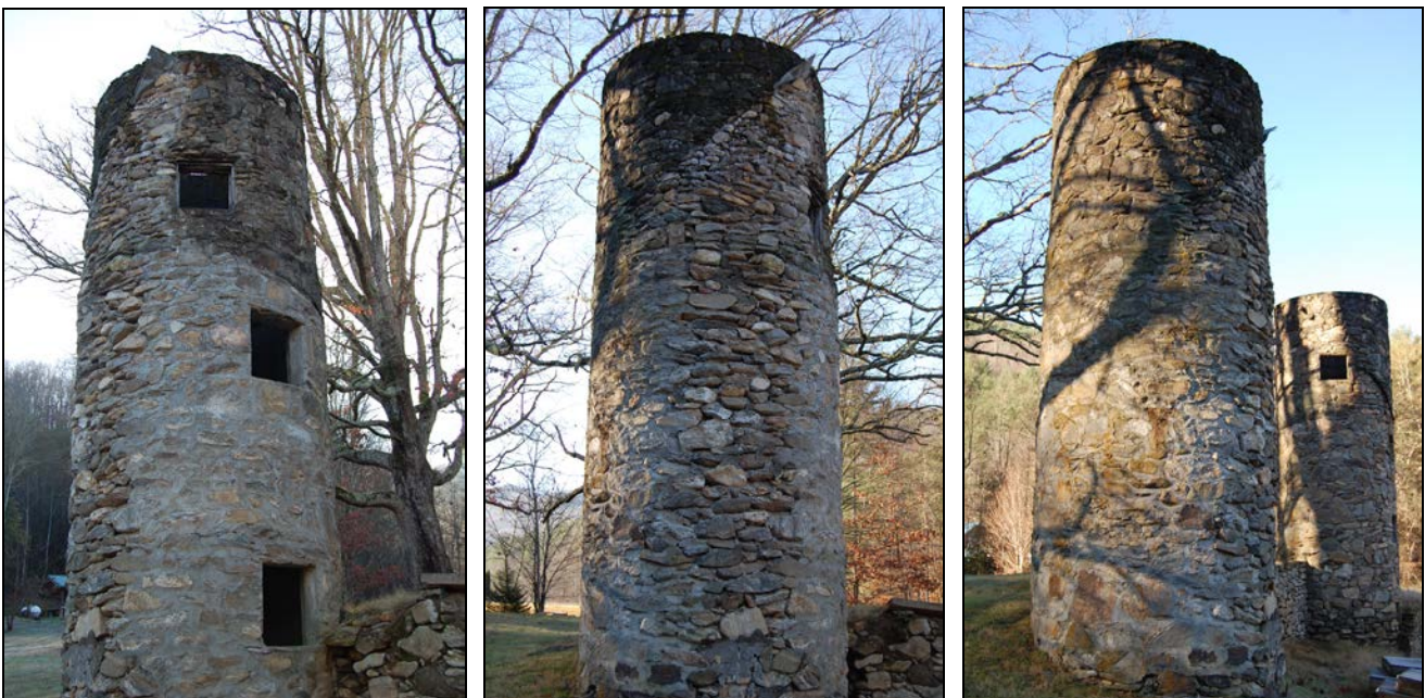
Figure 23. East Silo: west and northwest faces at left; north face at center; east face with west silo beyond at right
