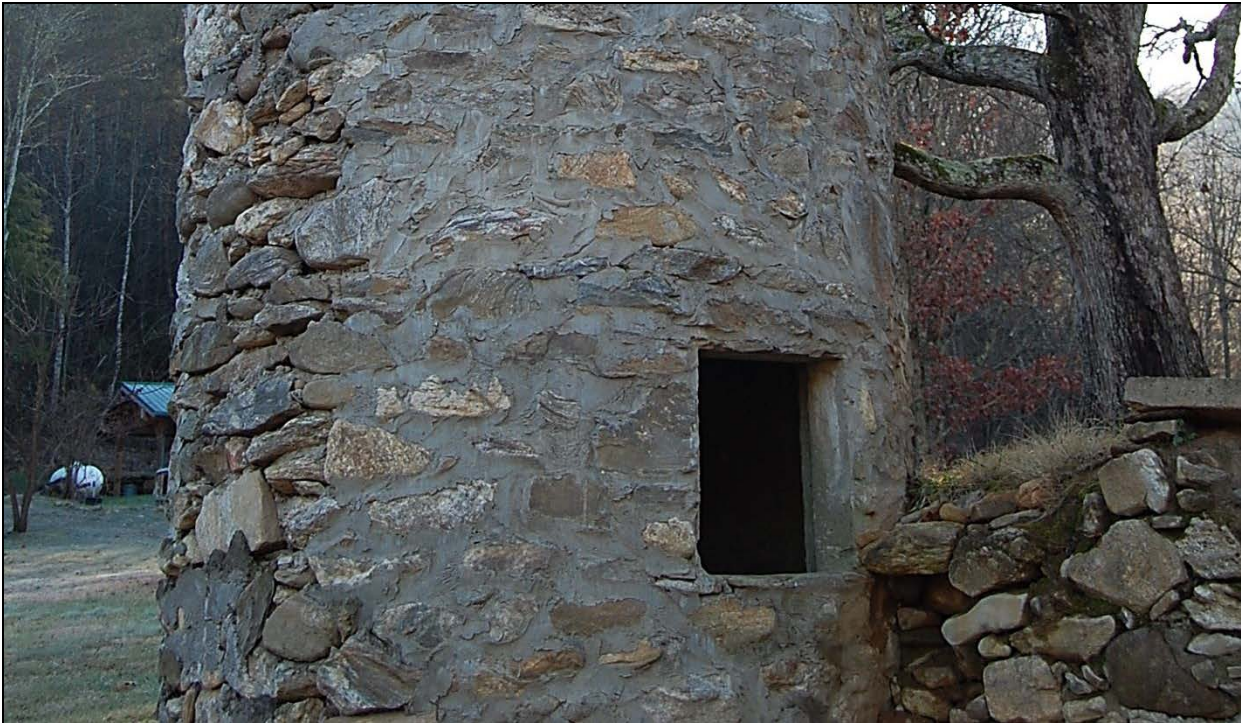
Figure 17. Looking southeast at point where south shed foundation wall abuts east silo
