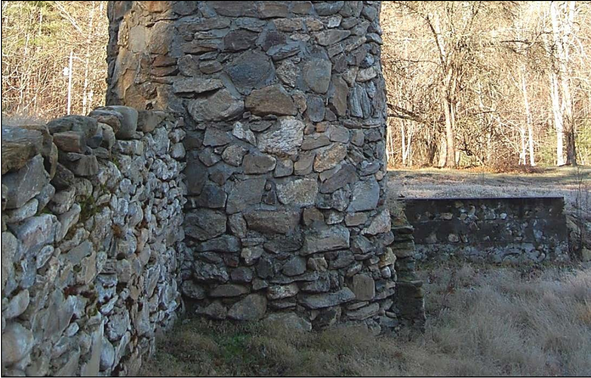
Figure 13. Looking west along south barn shed foundation wall, at left, to its abutting of west silo
