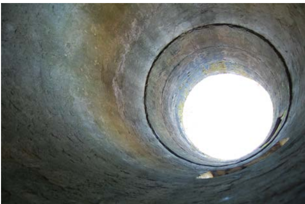
Figure 25. East Silo: interior cement surface
