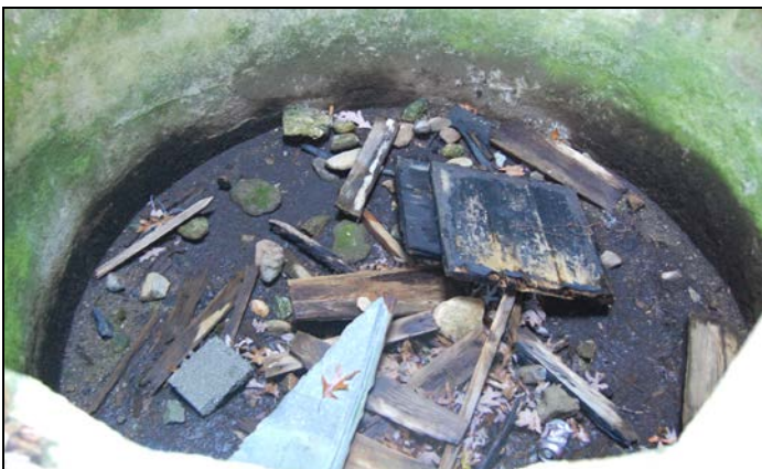
Figure 22. West Silo: silo floor with doors and other detritus
